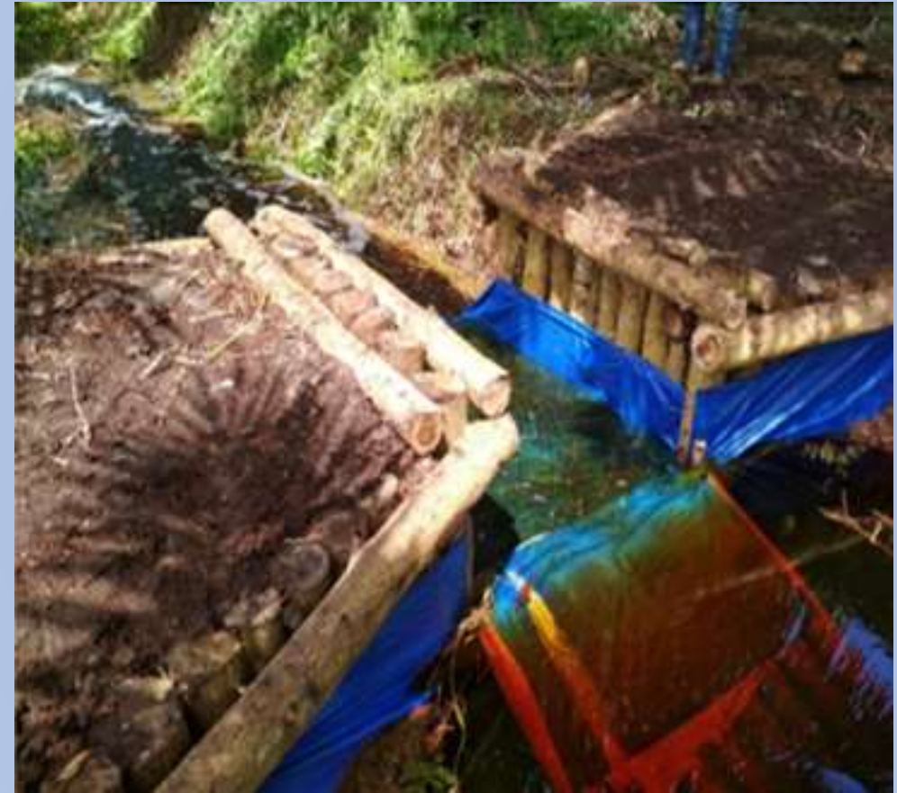
Construction of canal block in Wajok Hilir Village, Documentation on January, 2018
