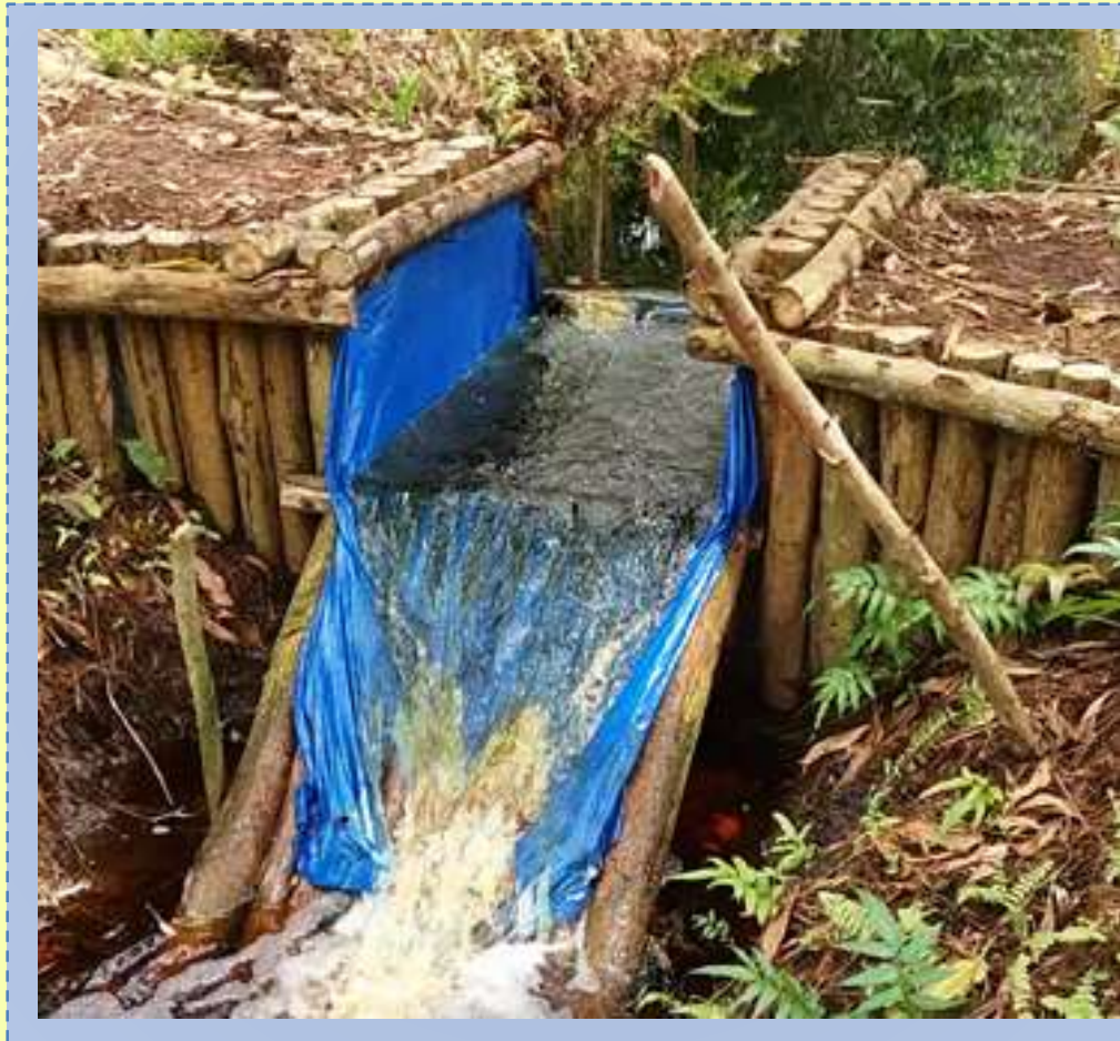
Construction of canal block in Wajok Hilir Village, Documentation on January, 2018
