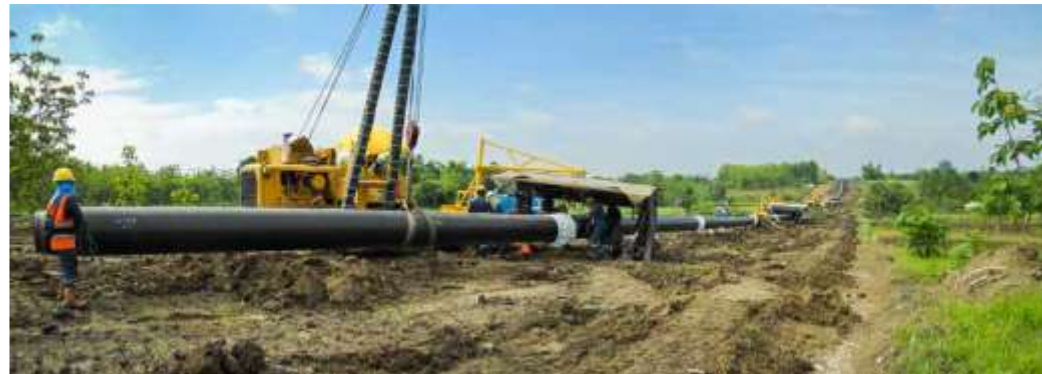
EPC-2: Onshore Pipeline
