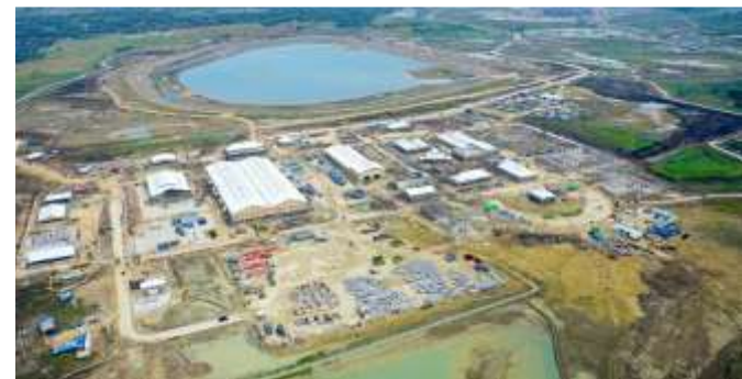
EPC-5 Infrastructure, Raw Water Basin and Flyover Road
