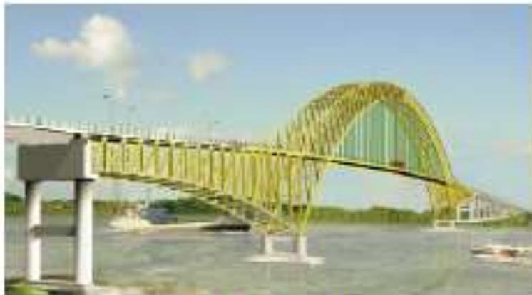
Teluk Mesjid Bridge
