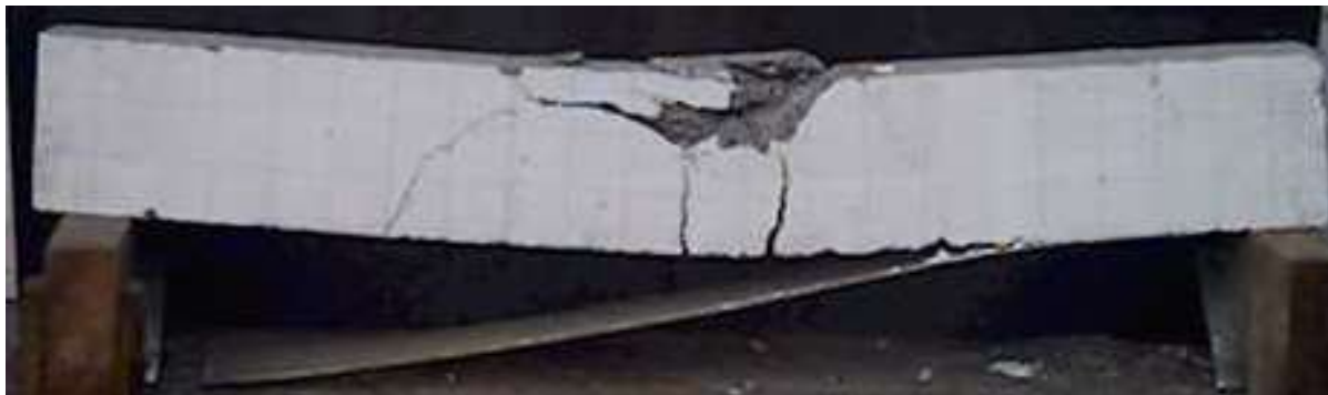
BS1: Beam with 2 layer GFRP, GFRP Debonding
