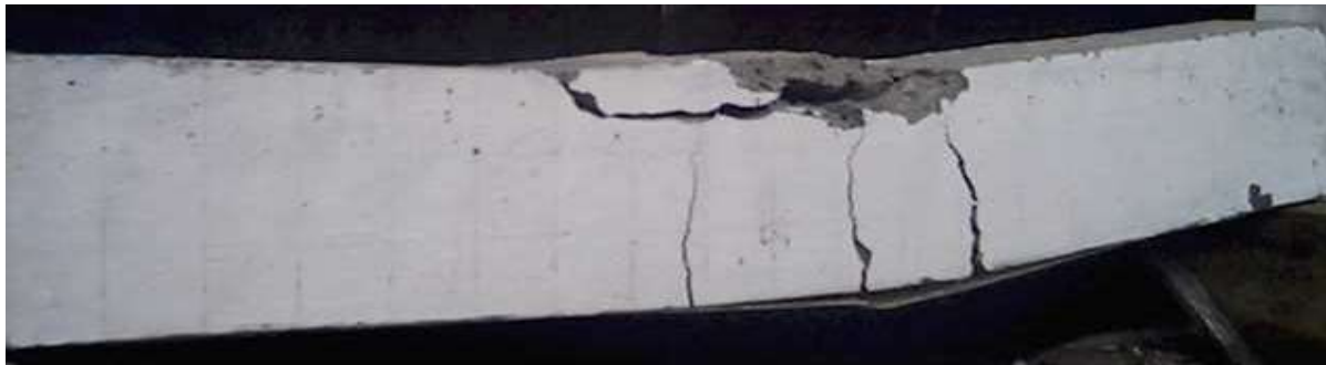
BS1: Beam with 1 layer GFRP, GFRP Rupture
